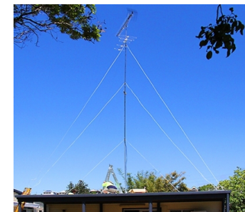
guy-wires supporting an antenna mast
