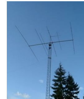
beam antenna atop an antenna tower
